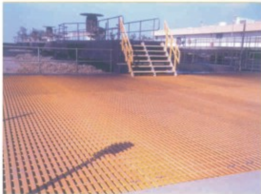
Pultruded Grating in Sewerage Treatment Plant
